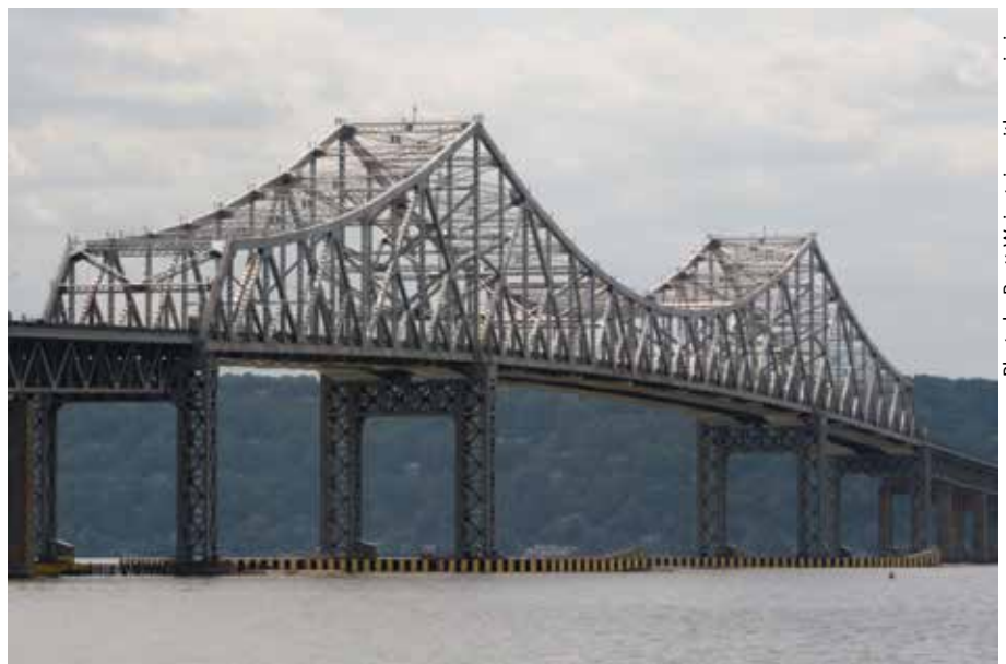
Figure 1. Tappan Zee Bridge, viewed from Tarrytown, New York.
